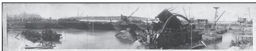
Figure 2 The cofferdam, Havana harbour, 1911
